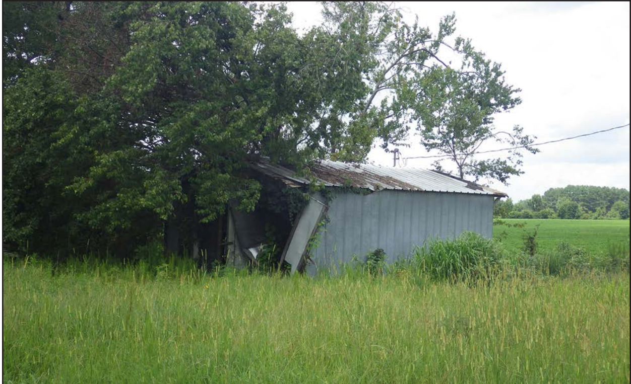
Photo 2. RIMG4212. CD1454, view of shed, facing northwest.
