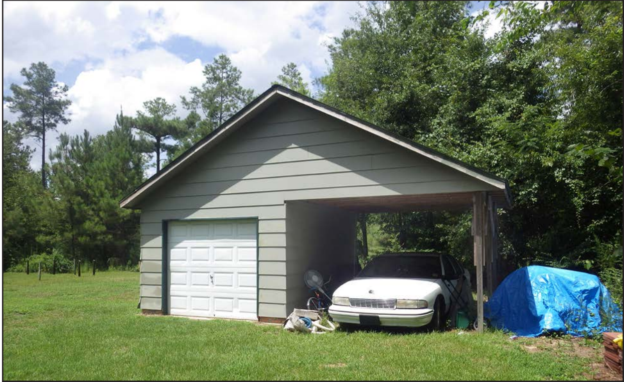
Photo 7. CD1456, view of garage, facing northwest.
