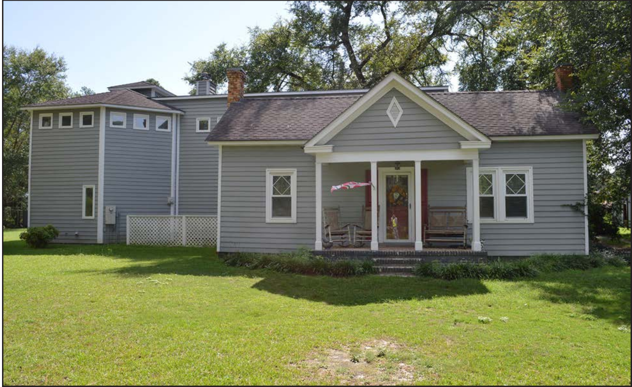
Photo 17. CD1459, facing southwest.
