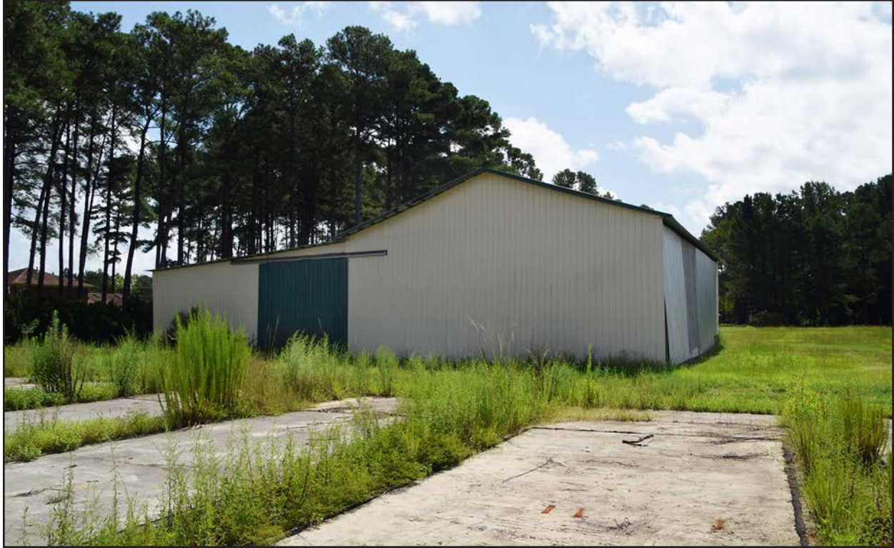
Photo 5. CD1455 barn and concrete foundations, looking east.
