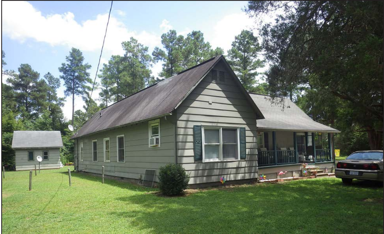
Photo 6. RIMG4216. CD1456, view of house and garage, facing east. .
