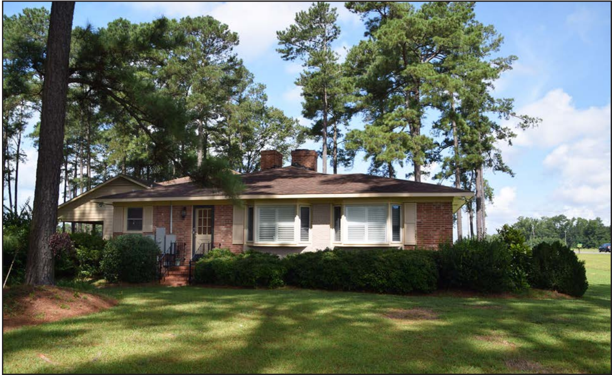
Photo 3. CD1455, looking west.
